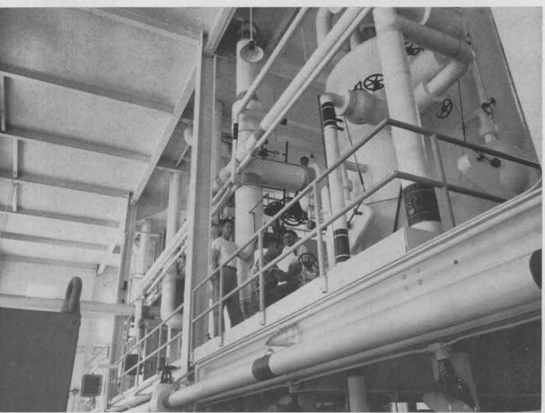
PREHEATING THE WATER that flows into the boilers is done at the top level of the plant with the large heating tank shown here. Air is also removed from the water in this heater. L to R are Elton Carroll, Homer Lawyer and Elbert Quail. William Dickens is behind the first group looking over a pipe.
